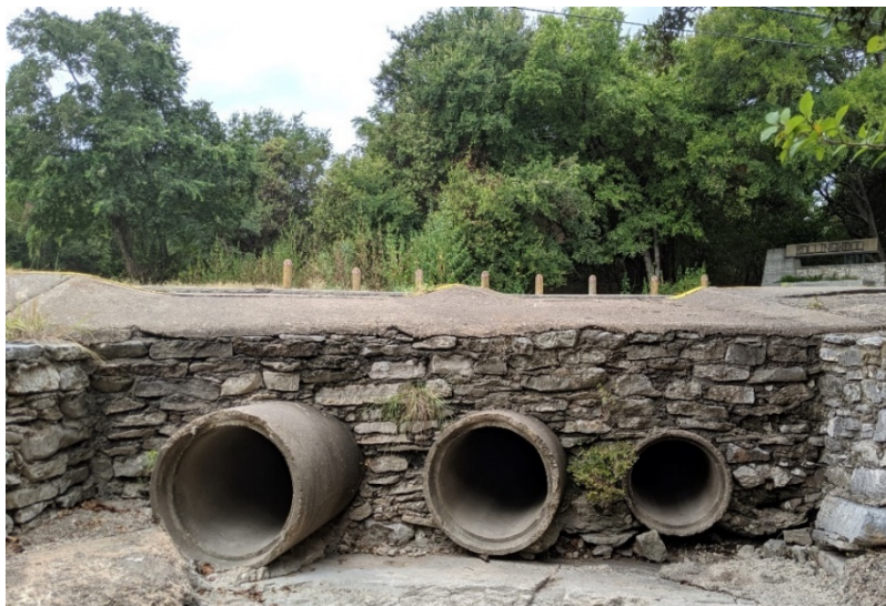
Figure 1: Edgegrove Drive Low Water Crossing (September 11, 2019)
