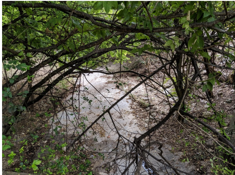
Figure 6: Rockway Cove Culvert, Looking Southwest/Upstream (September 11, 2019)
