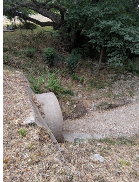
Figure 7: Pleasant Cove Culvert, Looking Northeast/Downstream (September 11, 2019)
