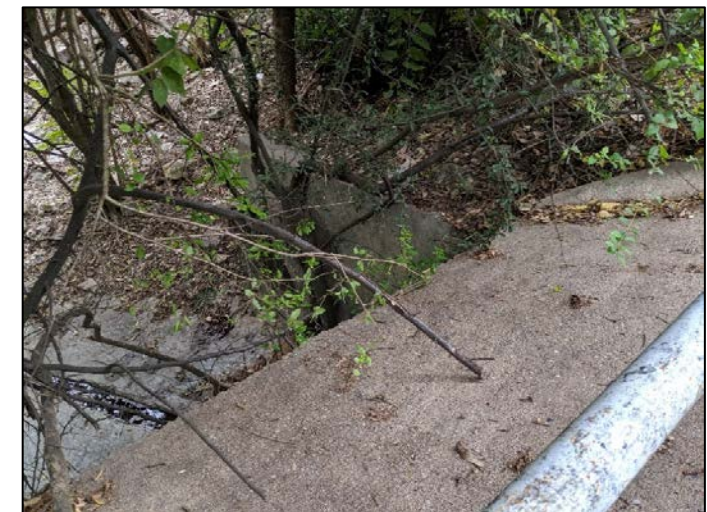
Outfall at Town Lake tributary. 09/11/2019
