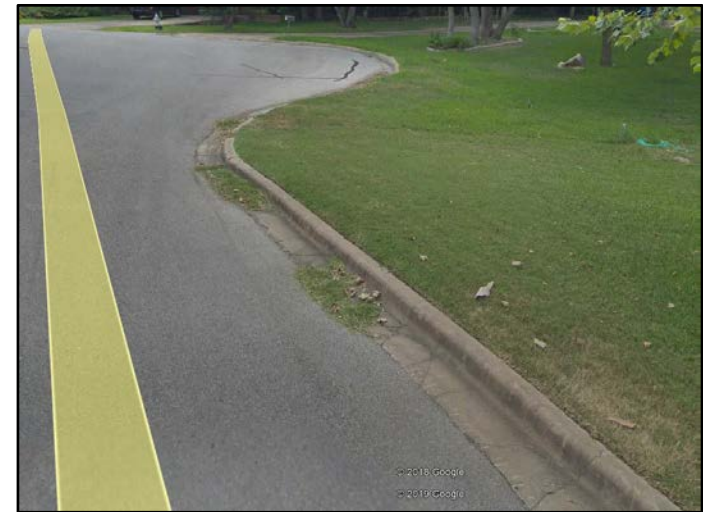
3 Randolph Place looking west.
