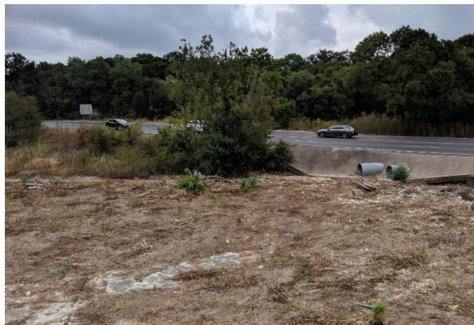
Figure 5: Bee Caves Road Culvert, Downstream (September 11, 2019)
