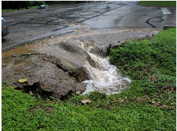
Figure 4: Nixon Drive Culvert, Looking Southeast/Downstream (June 6, 2019)
