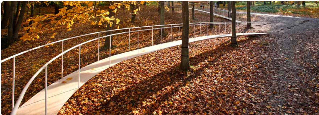
retaining wall + handrail
