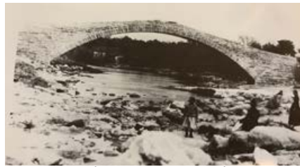
Stone Bridge Across Barton Creek 1880
