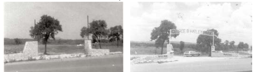
Erection of George B. Hatley Gate 1972
